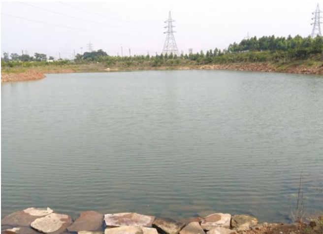
Digging of Ponds for Water Conservation
