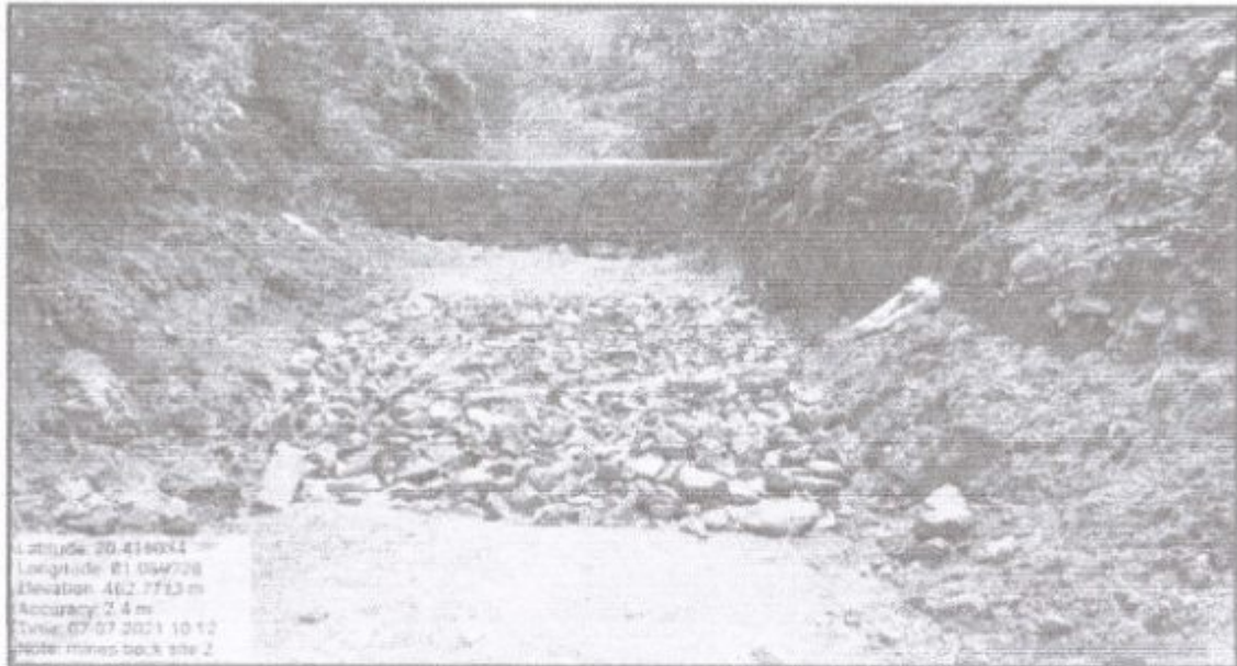
Structure 05: Recharge Well With Boulder Check Dams Latitude- 20.416034, Longitude- 81.059728
