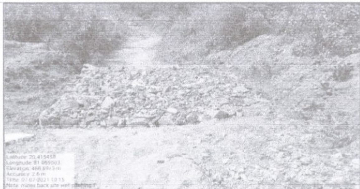
Structure 04: Recharge Well With Boulder Check Dams Latitude- 20.415458, Longitude- 81.059503
