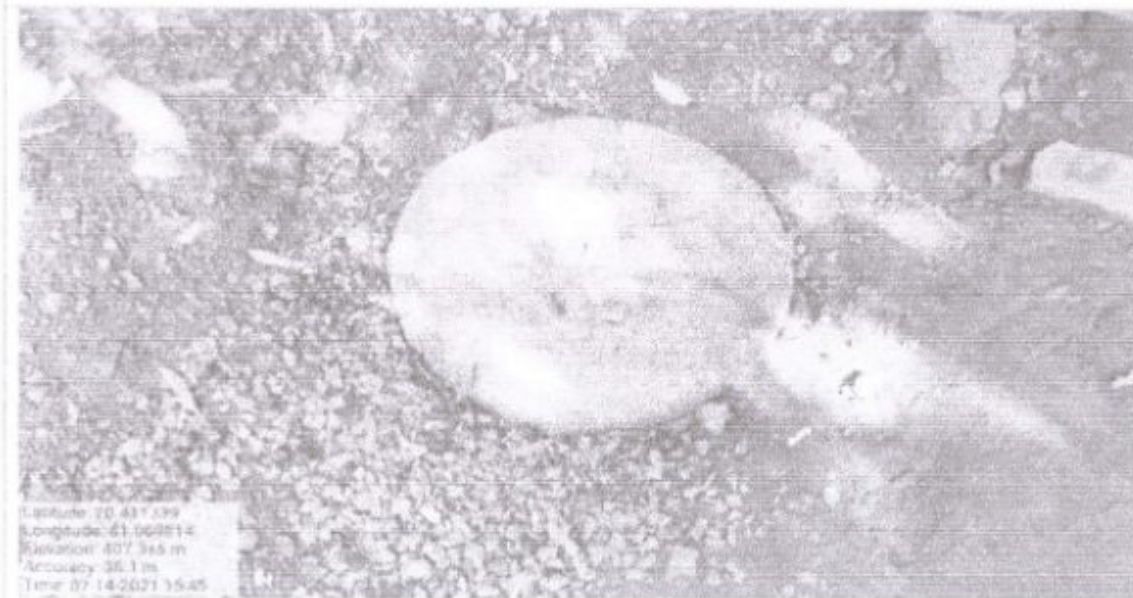
Structure 06 Recharge well 1 m dia 2 m depth
