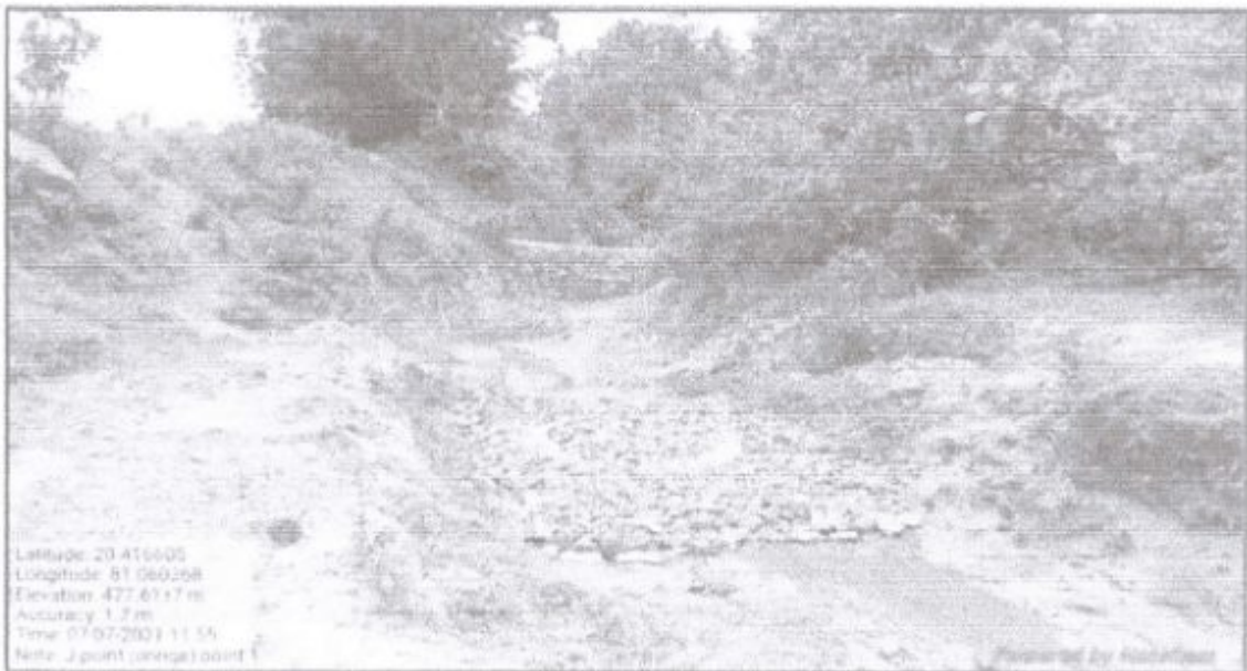
Structure 06: Recharge Well With Boulder Check Dams Latitude- 20.416602, Longitude- 81.060269
