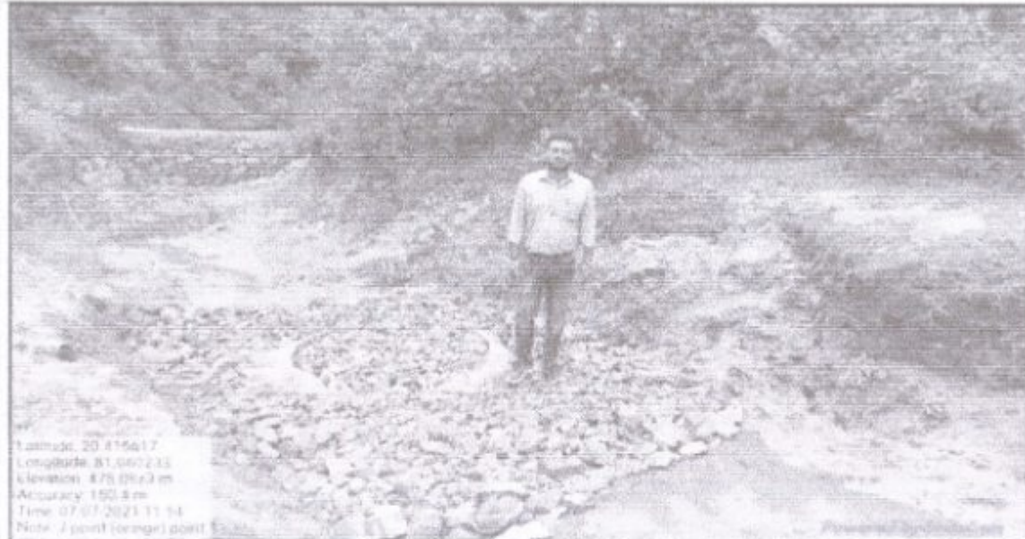
Structure 01: Recharge Well With Boulder Check Dams Latitude- 20.416617, Longitude- 81.060233
