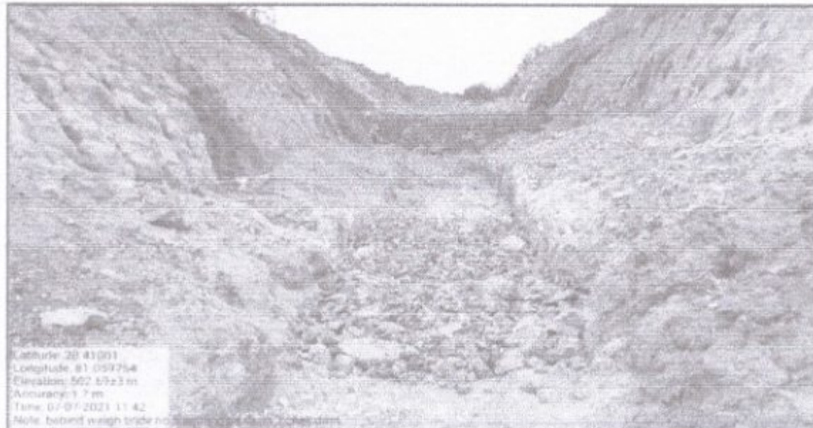
Structure 02: Recharge Well With Boulder Check Dams Latitude- 20.41001, Longitude-81.059754
