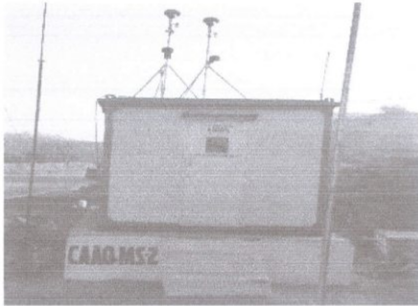
Continuous Ambient Air Quality Monitoring Station 2
