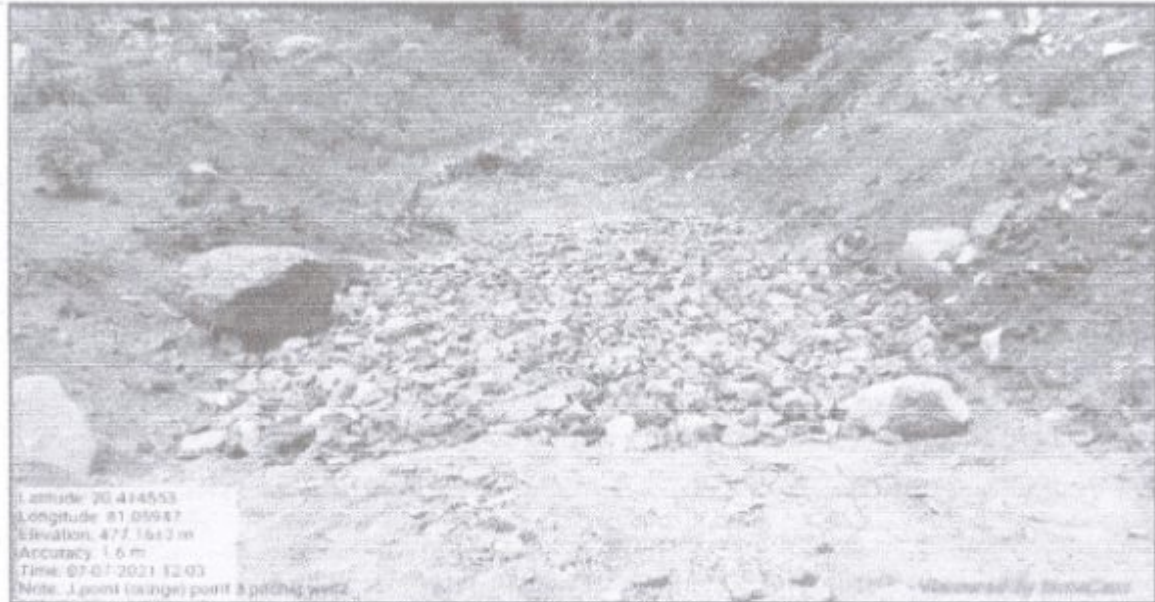
Structure 03: Recharge Well With Boulder Check Dams Latitude- 20.414553, Longitude- 81.059485
