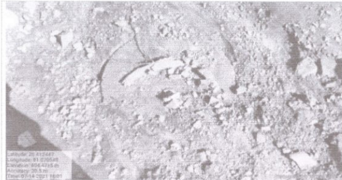
Structure 05 Recharge well 1 m dia 2 m depth
